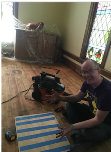
Robert Docker fixing the floor in the Altar area.
